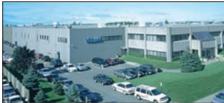
Montreal, Canada Velan Inc., Plant 2 and 7
