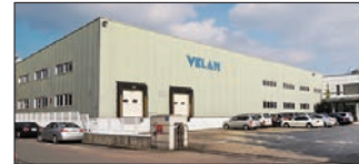
Ansan City, South Korea Velan Ltd., Plant 2
