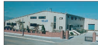
Ansan City, South Korea Velan Ltd., Plant 1
