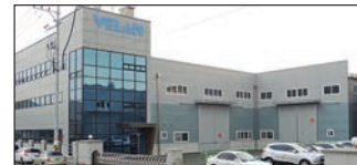
Ansan City, South Korea Velan Ltd., Plant 3
